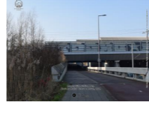
Crossing the tunnel
