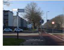
Residential buildings built on the 1960s
