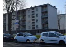
Residential buildings built on the 1960s
