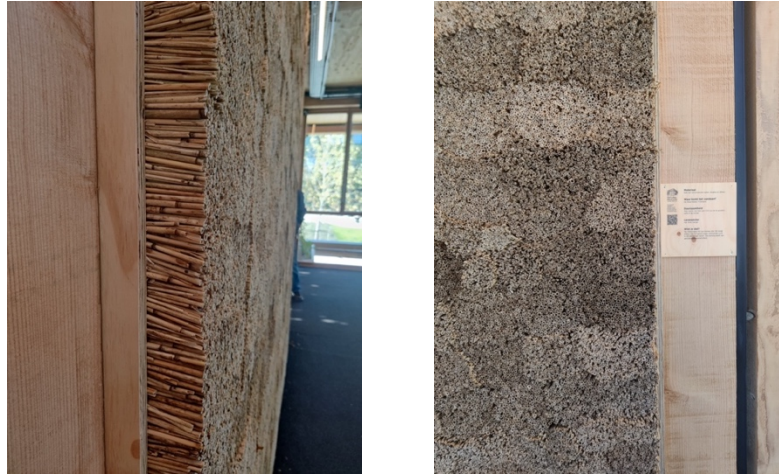
Figure 10. and Figure 11. Side and front view of reed wall in the natural pavilion, photographed by author, 13 October 2022
