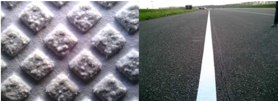
Figure 48: Location 10 ( 3M ESD ) application direction
