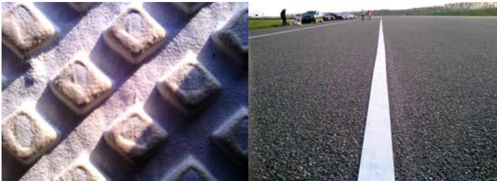
Figure 45: Location 8 ( 3M AW ) application direction
