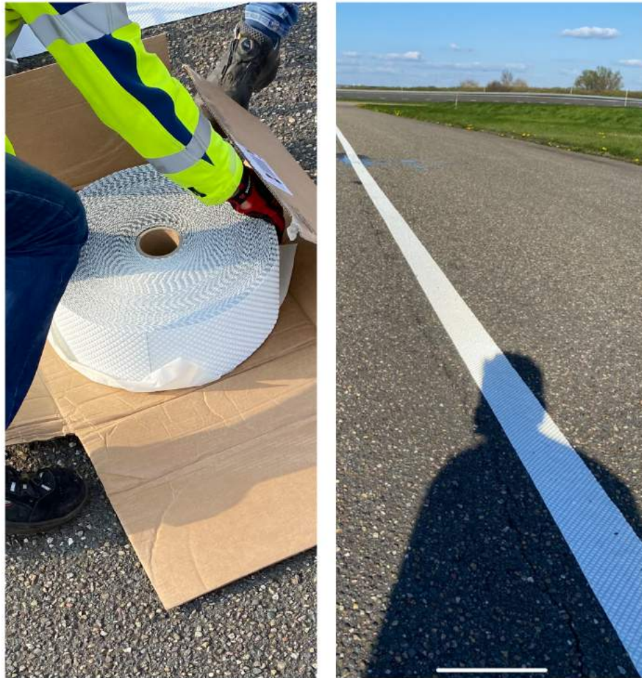
Figure 19: Left: 3M ESD tape roll unpacking ; Right: 3M ESD tape applied on test track
