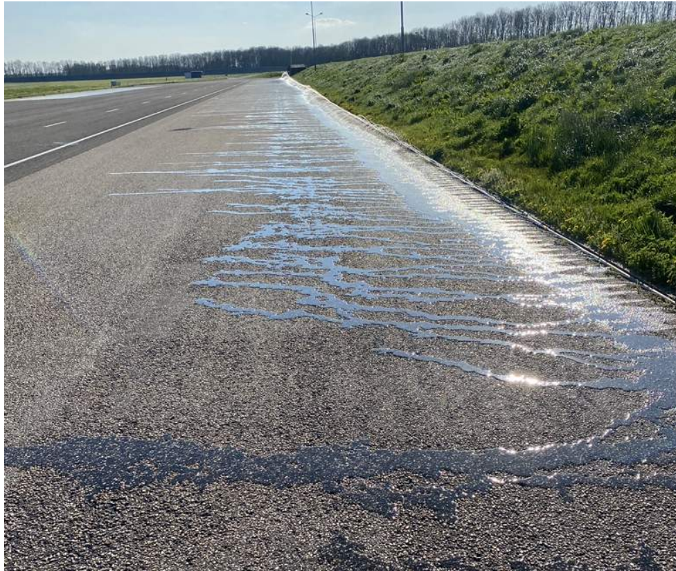
Figure 30: Water flowing onto the test track
