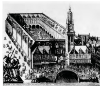
12.9 Amsterdam, Exchange, 1668-71, by Hendrik de Keyser
