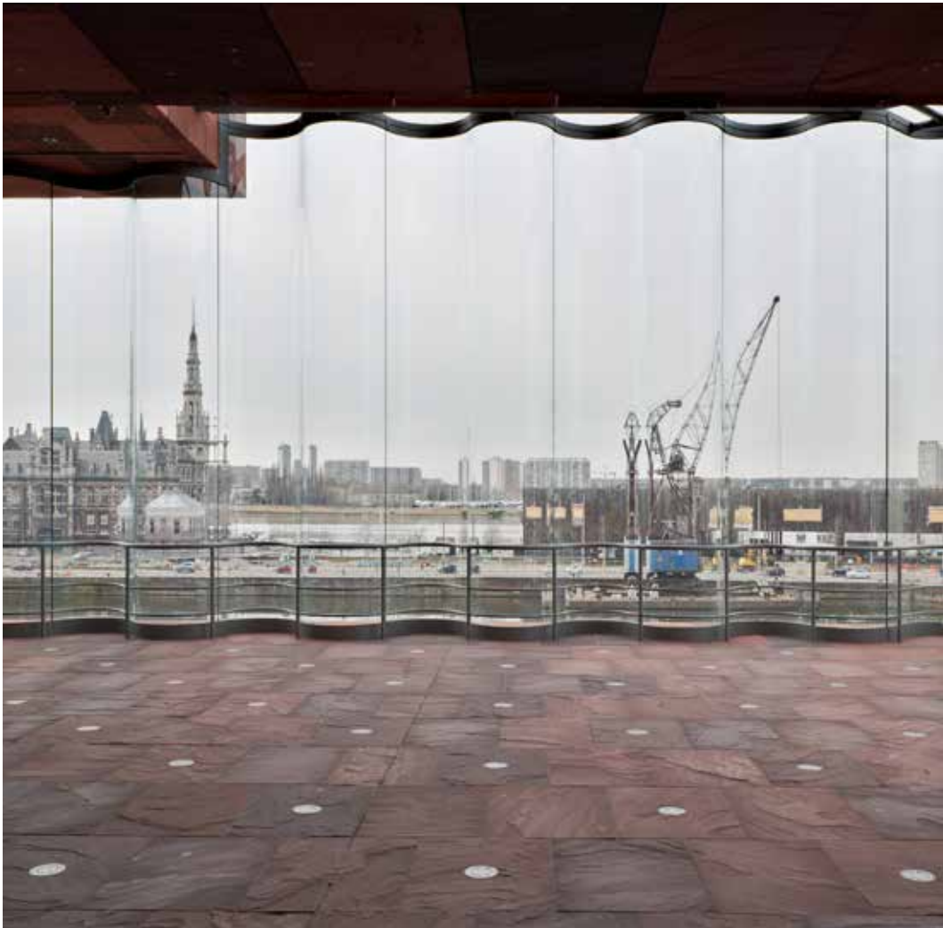
FIG. 5.31 View through the curved glass in the MAS Museum (Antwerp, BE). Source: https://commons.wikimedia.org/wiki/File:Curved_glass_as_seen_from_inside_the_MAS_museum_(Antwerp,_BE).jpg . https://upload.wikimedia.org/wikipedia/commons/9/9d/Curved_glass_as_seen_from_inside_the_MAS_museum_%28Antwerp%2C_BE%29.jpg . Trougnouf [CC BY-SA 4.0 ( https://creativecommons.org/licenses/by-sa/4.0 )]
