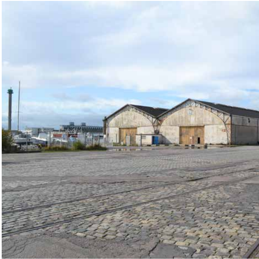
FIG. 5.59 Old port warehouses
