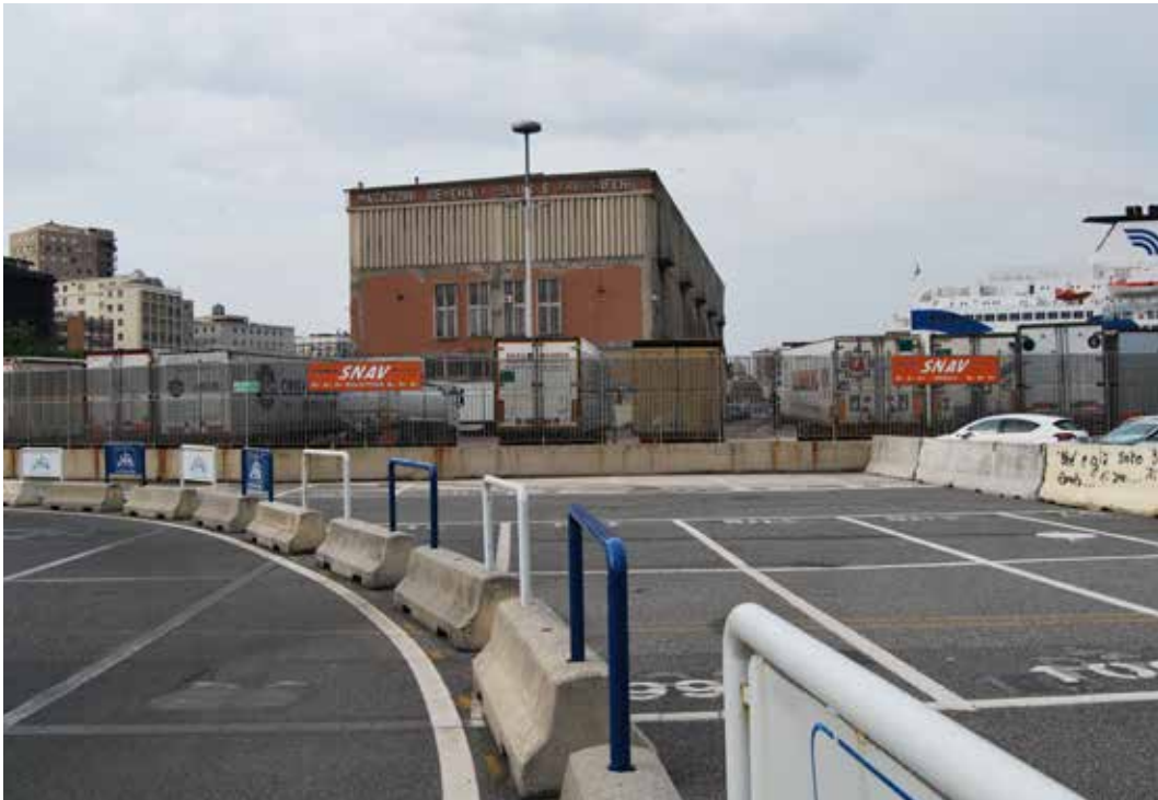
FIG. 4.8 "Magazzini Generali" building.
