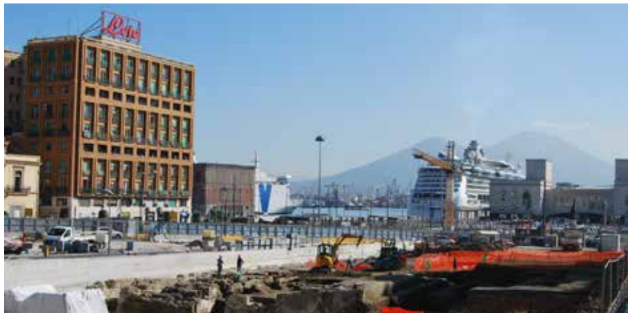
FIG. 3.4 Municipio square. The excavations for the metro station.
