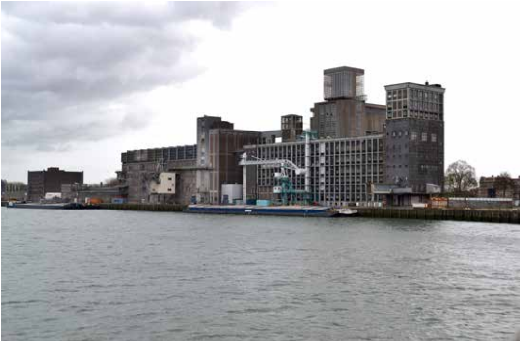
FIG. 5.16 Codrico building, Rijnhaven area, 2016
