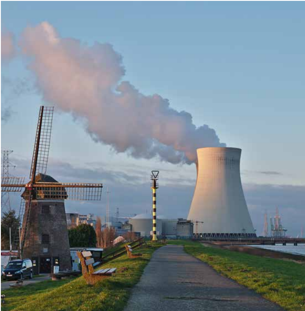
FIG. 5.48 Doel village. Source: https://commons.wikimedia.org/wiki/File:De_Molen_(windmill)_and_the_nuclear_power_plant_cooling_tower_in_Doel,_Belgium_(DSCF3859).jpg . Trougnouf, CC BY-SA 4.0 < https://creativecommons.org/licenses/by-sa/4.0/ >, via Wikimedia Commons
