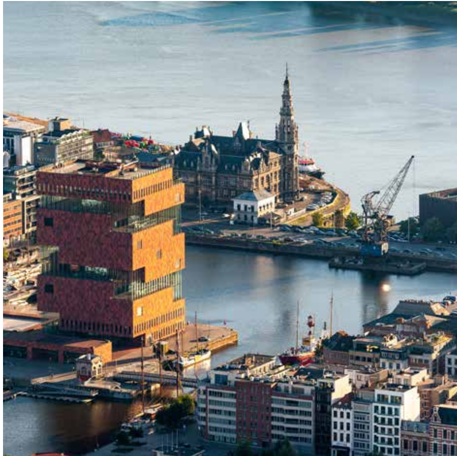
FIG. 5.44 MAS museum at the Bonapartedok._Source: ©Gianni Camilleri_Neutelings Riedijk Architects_kl
