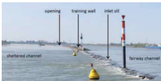
Figure 3. Inlet sill at upstream end of the longitudinal training wall at Wamel.
