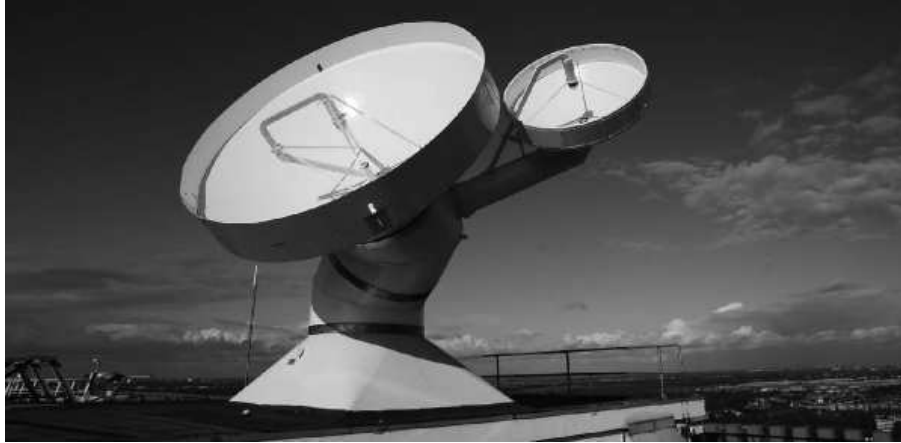
Figure 4.8: Layout of the PARSAX radar on top of the Faculty of Electrical Engineering, Mathematics and Computer Science [37].
