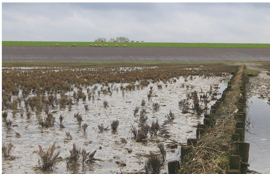
Figure 1.3: Brushwood dams to create artificial shelter of salt marsh vegetation from waves and currents. The dike is visible in the background (Photo: V. Vuik).
