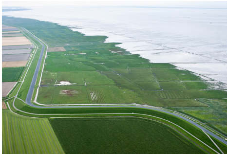
(c) Groningen, salt marsh, Wadden Sea. Marsh elevation 2.0 m+NAP, width 800 m, slope 1:750. Dike height 9.1 m+NAP, slope 1:4. Design conditions: h = 5.3 m+NAP, H_{m0} = 1.8 m, T_{m-1,0} = 5 s.
