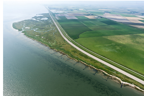
(d) Texel, salt marsh Schorren, Wadden Sea. Marsh elevation 1.8 m+NAP, width 400 m, slope 1:250. Dike height 6.9 m+NAP, slope 1:3. Design conditions: h = 4.4 m+NAP, H_{m0} = 1.4 m, T_{m-1,0} = 5 s.
