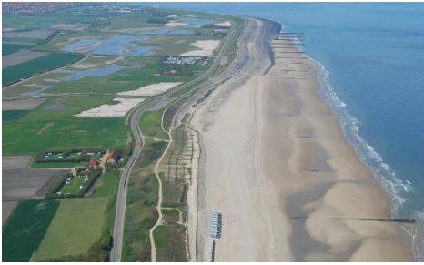
(a) Westkapelle, sandy foreshore, North Sea. Foreshore elevation 4.0 m+NAP, 1:40 slope. Dike height 12.6 m+NAP, 1:6 slope. Design conditions: h = 4.9 m+NAP, H_{m0} = 4.6 m, T_{m-1,0} = 9 s.
