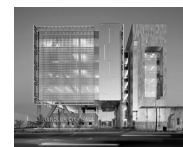
Chandler Town Hall
