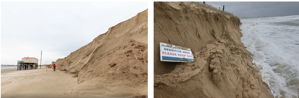
Figure 1.1: Severe dune erosion and subsequent dune foot repositioning. (left) Banjaardstrand, NLD. Photo from Adriaansens (2022) (right) Elouera Beach, AUS. Photo from Trembath (2020).
