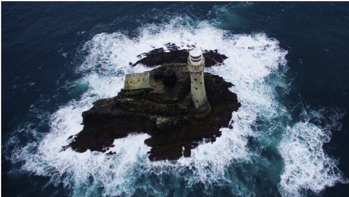
Fig. 1. Drone image of Fastnet lighthouse collected during the field modal test by Mr. James Bassitt (University of Exeter).
