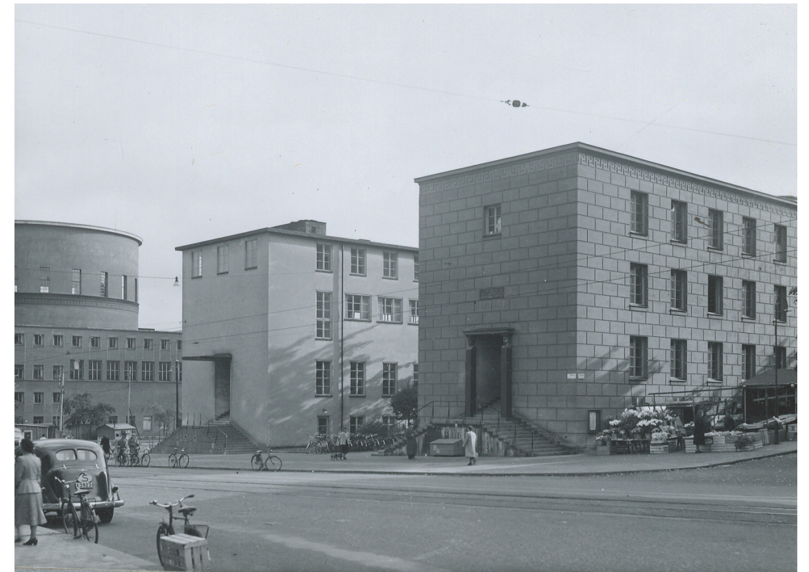
Archival Photograph View to the library from Odengatan, 1948
