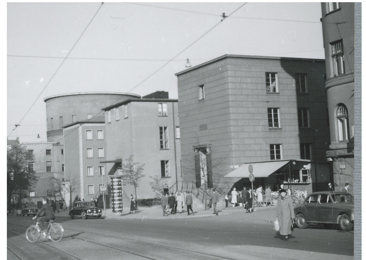
Archival Photograph View to the library from Odengatan, 1956
