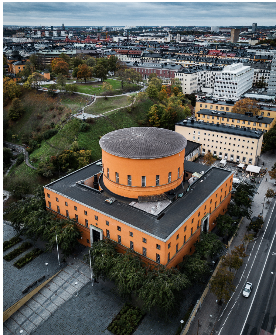
Photo Bird eye perspective on the Stockholm city library, with the 3 annex buildings.
