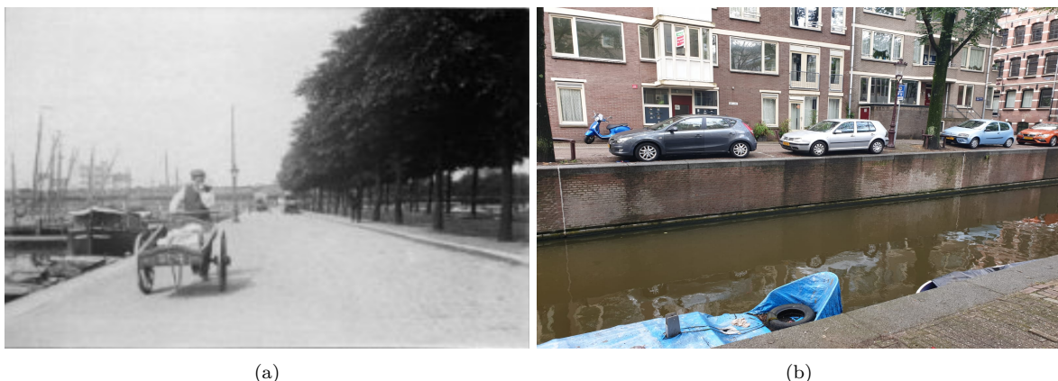
Figure 1.1: The difference in how quay walls were used 100 years ago (a) and nowadays (b).
