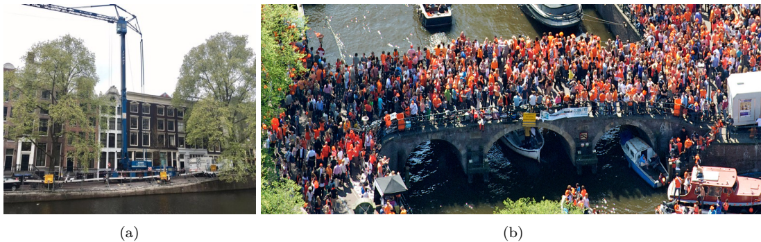
Figure 2.7: Two types of extra temporary loads acting on the quay walls: (a) heavy cranes, (b) large crowds during Kingsday.
