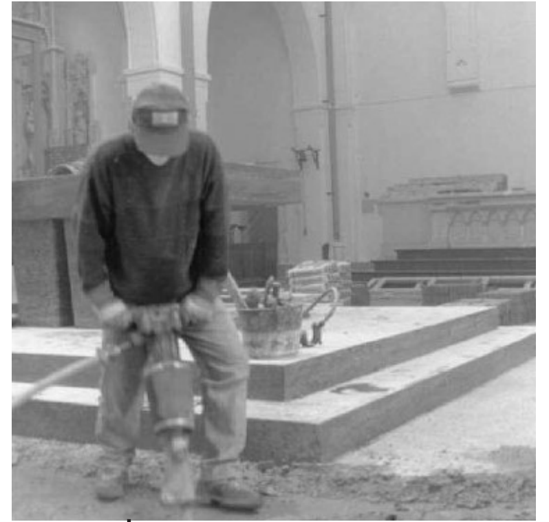
ground floor is replaced
