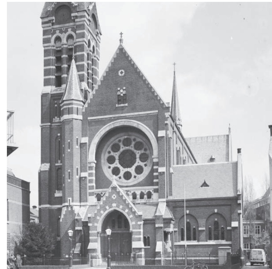
Detailed facade towards the market square
