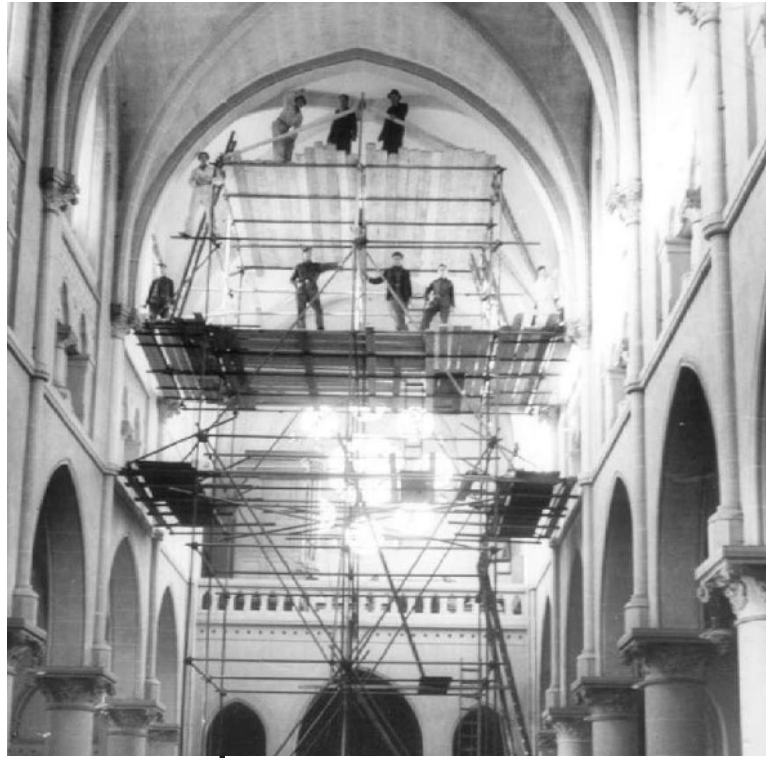
interior is painted over
