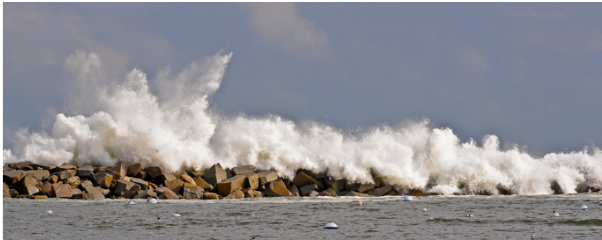
Figure 1.1: Wave overtopping of a breakwater (credits: Liz Mackney)
