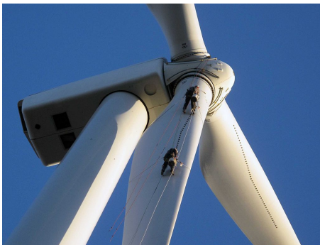
Figure 1.1: Installation of vortex generators on a wind turbine (©Robert Bergqvist)
