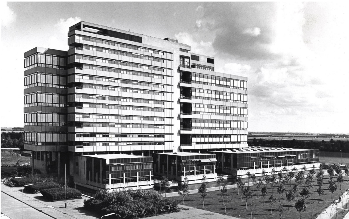
Figure 2: Broekbakema, exterior photo of Faculty of architecture and the Built environment in TU Delft, 1970 (Broekbakema)
