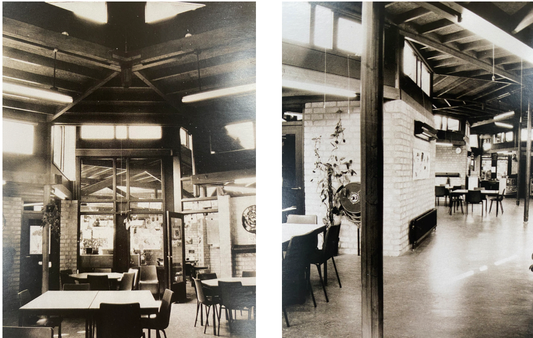
Figure 9: Jan Verhoeven, Timber structure in Basisschool Airborne (Zahle, Mette. 2012)
