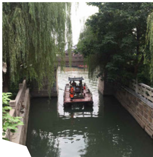
FIG. 3.23 Salvage garbage and remove silt manually 人工打捞垃圾、清除淤泥
