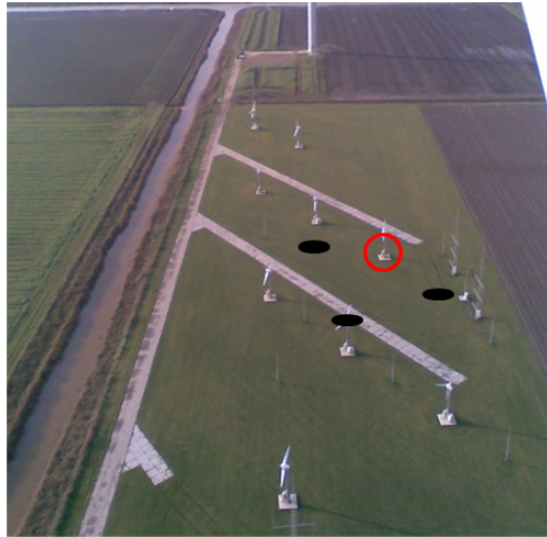
(a) Scaled wind farm layout with turbine under test (red circle) and indicated scanner positions (black dots)
