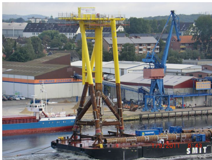
Figure 3.4: Twisted Jacket for the wind farm Hornsea
