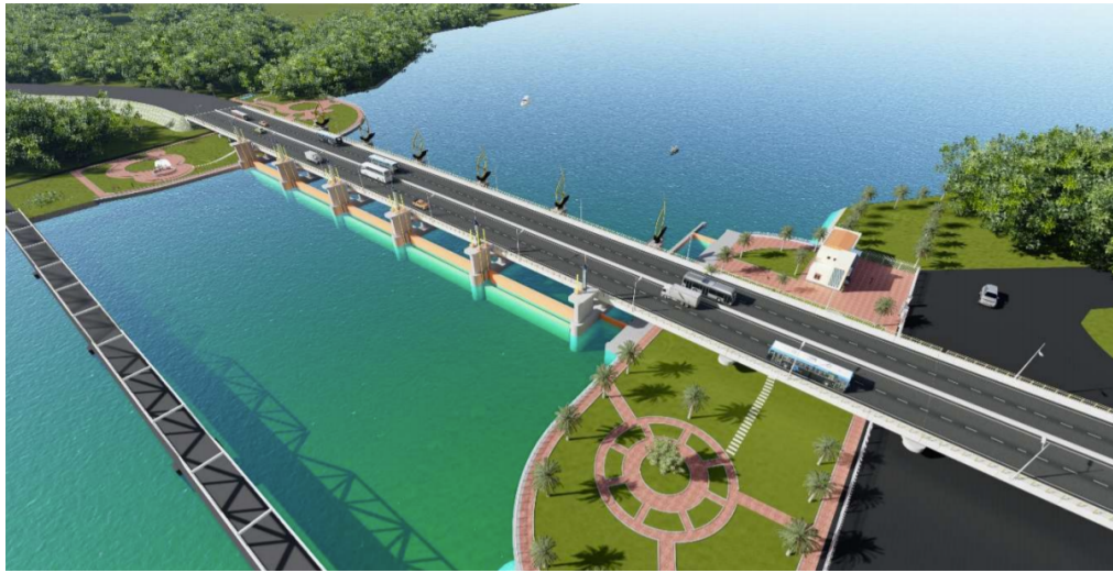
Figure 3.6: An Impression of the Saltwater Intrusion Dam at Nha Trang. [39]
