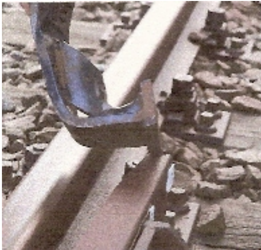
Figure 36. The dropped right-hand catcher striking a check rail (reconstruction)
