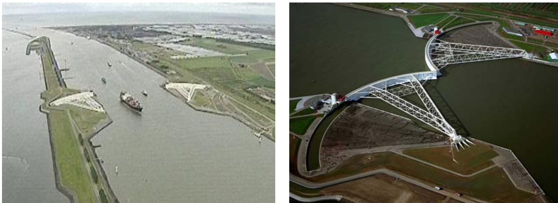
Figure 11. Maeslant Barrier in normal position (left) and closed position (right). Its design was dictated by the need to comply with a preset risk estimation.
