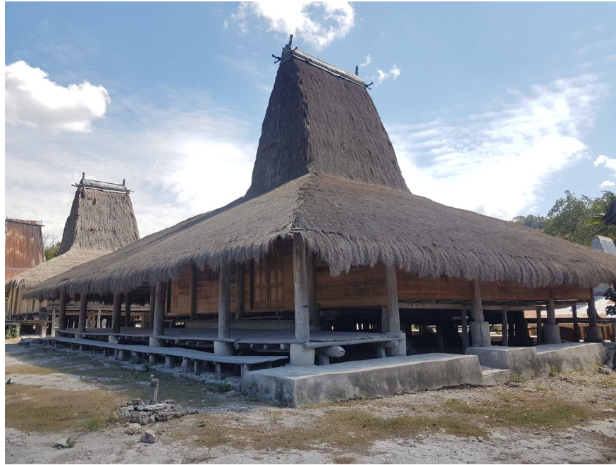
Figure 34: Traditional Sumbanese House
