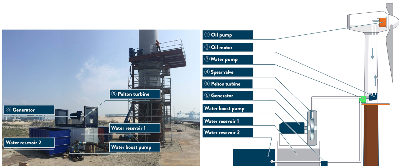
Figure 3. Overview of the intermediate DOT500 hydraulic wind turbine configuration. An oil pump is coupled to the rotor low-speed shaft in the nacelle and hydraulically drives an oil motor in the bottom of the tower. This closed oil circuit serves as a hydraulic gearbox between the rotor and water pump. The motor is mechanically coupled to a water pump, which produces a pressurized water flow. The flow is converted to high-velocity water jets by spear valves and a Pelton turbine–generator configuration harvests the hydraulic into electric energy.
