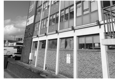
Closed-off plinth and uniform facade
