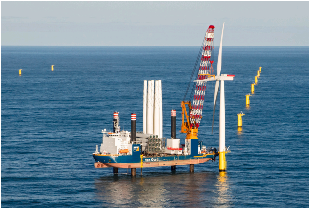
Fig. 1. Aeolus offshore wind turbine installation vessel (courtesy of Van Oord).
