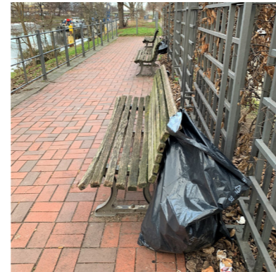
[Fig. 16] Lacking maintenance
