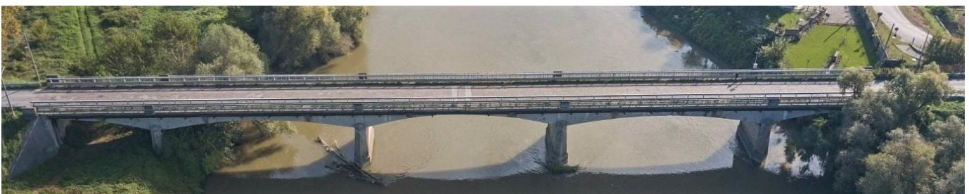
Figure 2 The Marcaria Bridge.
