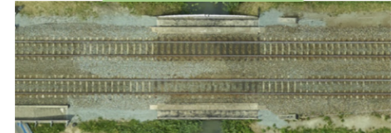
Aerial Photo of B4
