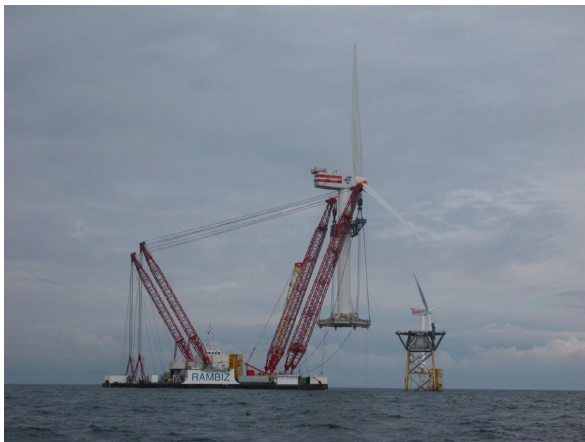
Figure 2.4: Transport and Installation of two 5MW Wind Turbine Generators for the Beatrice Demonstrator Project.
