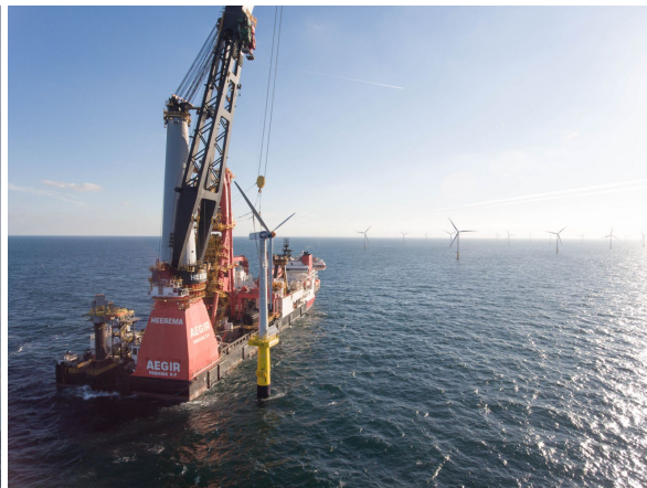
Figure 2.5: Installation of the first offshore WTG with a slip joint by floating heavy lift vessel, the Aegir.
