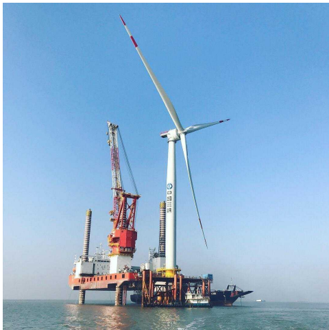
Figure 2.9: Installation of 6MW turbine for the Xinghua Gulf demo project.
