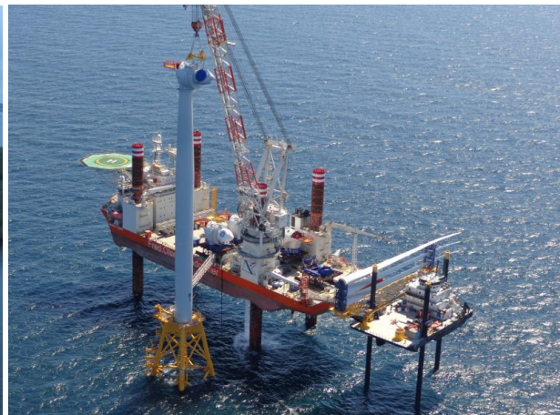
Figure 2.8: Brave Tern installing a nacelle for the Block Island wind farm.
