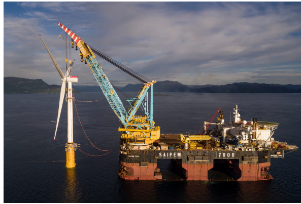
Figure 2.6: Saipem 7000 installing a 6 MW inshore wind turbine on a floating substructure.
