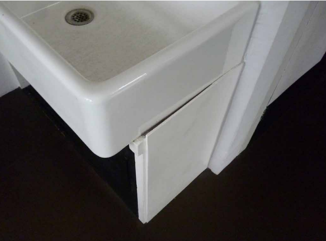
FIG. 5.2 Deformation of thin timber elements of furniture
