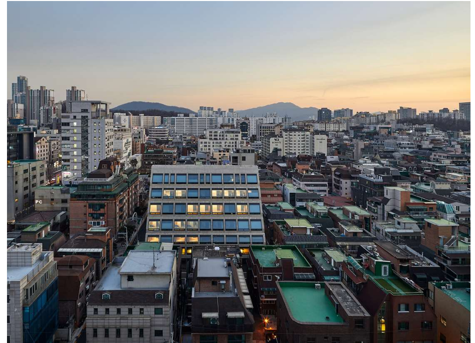
Fig. 11. Slanted windows give apartments great views, while maintaining privacy. (c) Rohspace (Archdaily, 2021)
