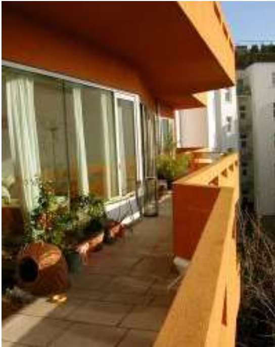
Fig. 95. Gallery also serves as an outdoor space (c) Harald Huscava, 2008
