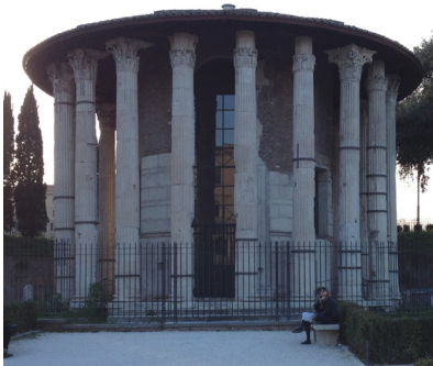
3 Tempio di Ercole Vincitore in Rome, 18 th century and today. Later attachments are demolished.
