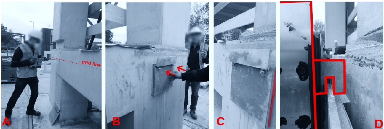
Figure 81: Steps for the placement of the modules on the concrete structure
