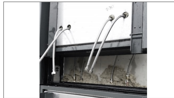
Figure 101: The flexible pipes that were connected just before the placement of the facade modules.
