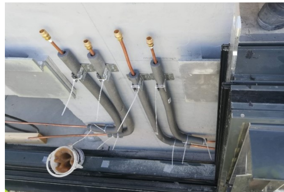
Figure 101: The flexible pipes that were connected just before the placement of the facade modules.
