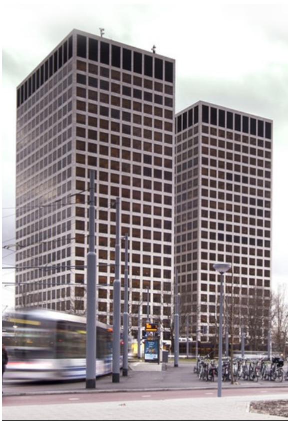
Figure 73: Europoint Towers, Rotterdam
