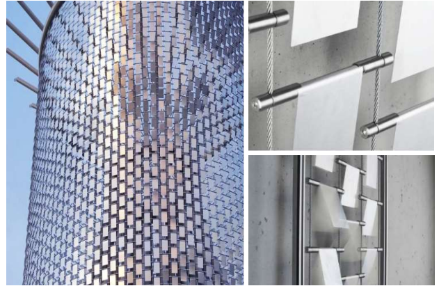
Figure 11: Wire Rope in Façade, Source (BuildingandInteriors, 2019)
