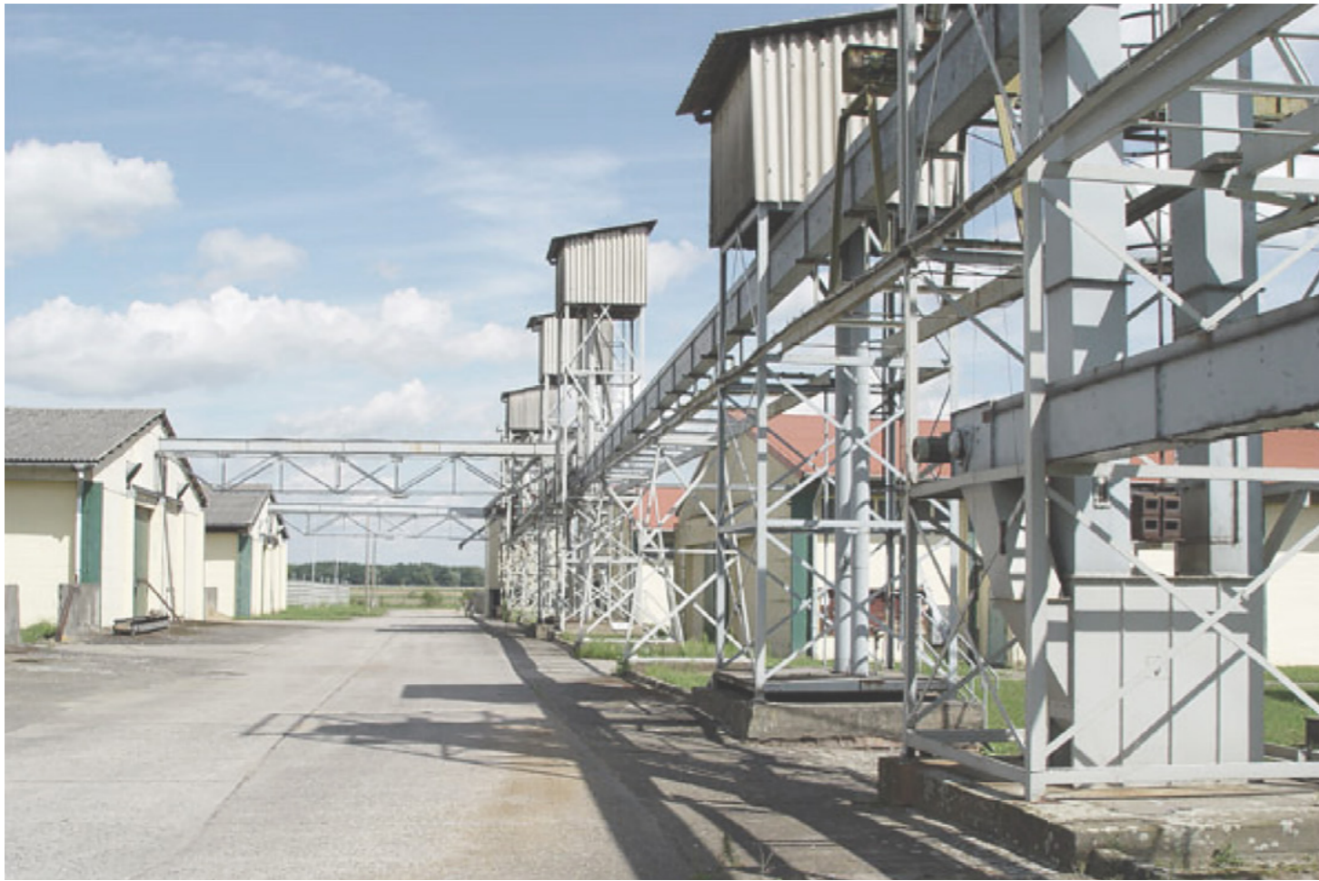
Fig. 6.6.1 Impression from site of feed processing plant. Source: www.landhandel-luckau.de
