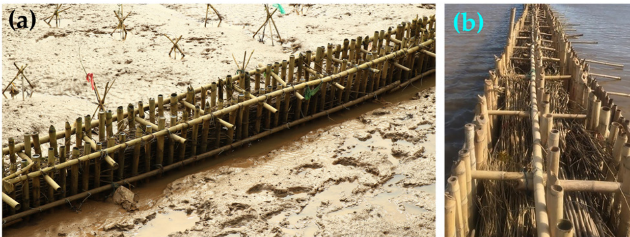
Figure 1: Type of bamboo fences in the Mekong Delta. Courtesy Hoang Tung Dao, 2016 (a) and Le Xuan Tuan, 2020 (b).
