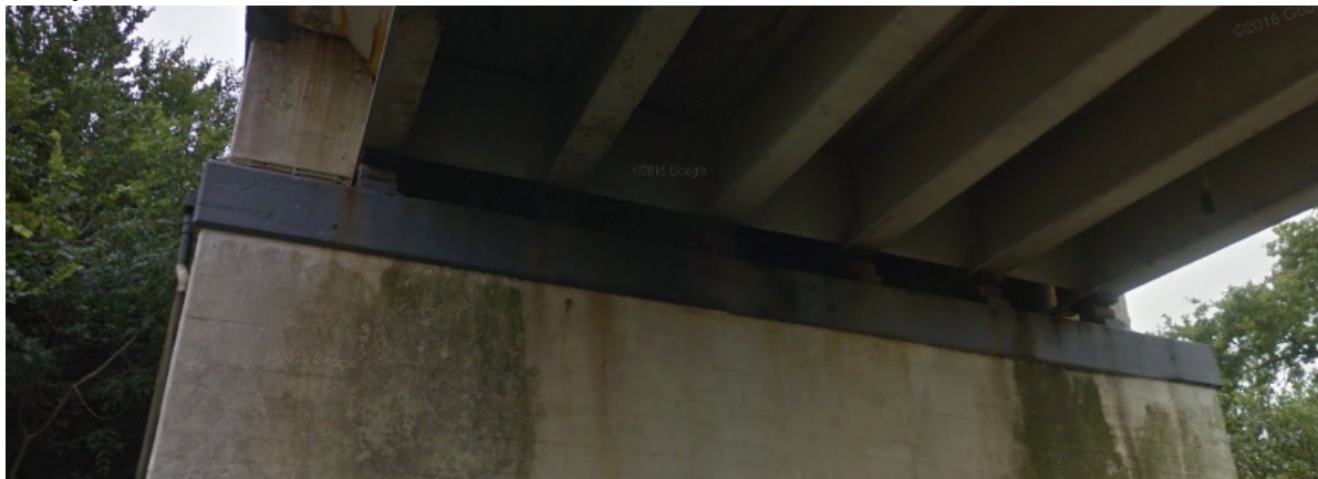
(b) Picture of the bridge.
