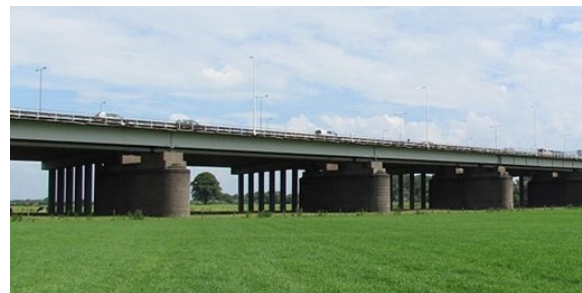
(b) IJsselbrug A12 (girder bridge).
