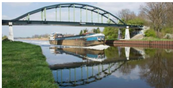
(a) Leemslagenbrug (arch bridge).
