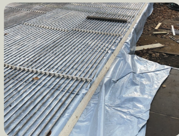
Image 90: Finish of plastic sheet with wooden strip.
