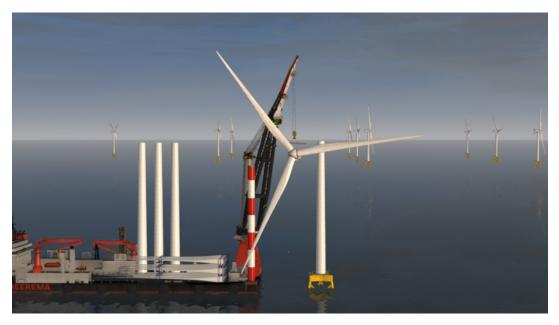
Figure 2.1: Lifting the RNA from the assembly tower to the WTG tower.
