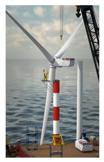
Figure 1.7: Lifting the RNA from the assembly tower on deck of the installation vessel to the already installed tower.
