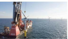
Figure 1.6: Aegir from Heerema Marine Contractors (monohull) installing the DOT offshore wind turbine (HMC).
