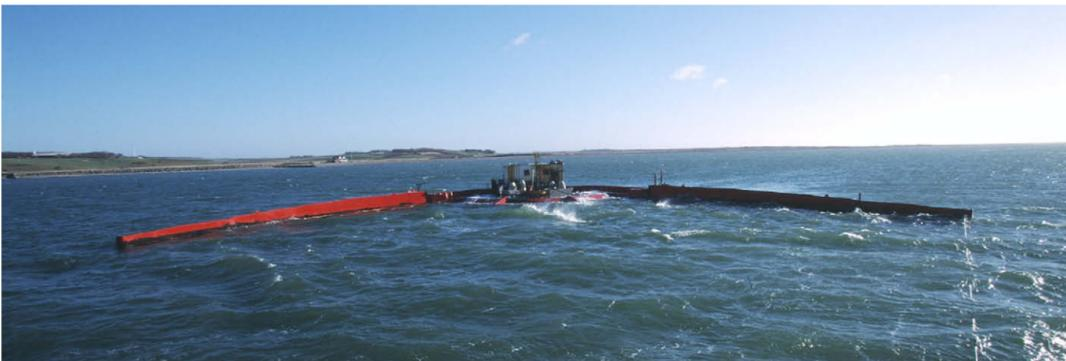
Figure 2.3: The Wave Dragon overtopping wave energy device. This image has been taken from Tedd and Kofoed [19].
