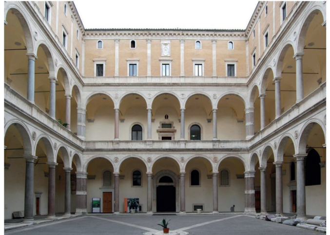
Figure 14: Right, Courtyard of Palazzo della Cancelleria, Rome, Italy. Image from Waters, Reviving Antiquity with Granite , 160.
