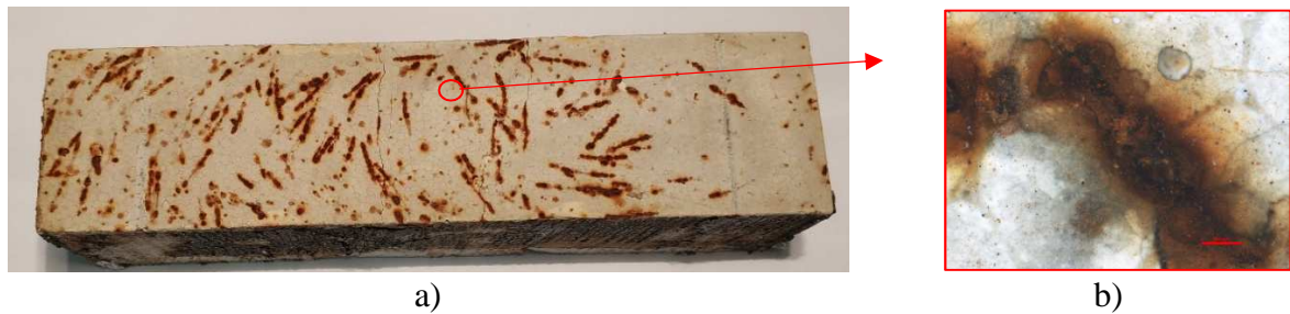
Figure 5: a) Exposed specimen surface after wet-dry cycles; b) Detail of fibre corrosion on specimen surface.
