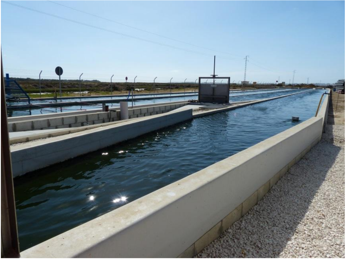
Figure SI-2: Photo and layout drawing of the HRAP WW treatment plant in Almería, Spain
