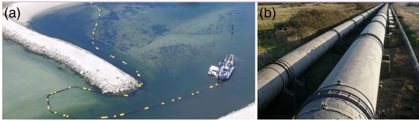
Figure 1.2: (a) Transport of sediments from a dredger via horizontal pipelines over water using flotation buoys (damen.com). (b) Slurry transport pipelines (fluidflowinfo.com).
