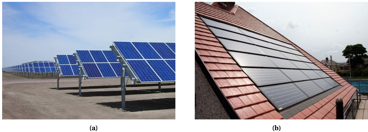
Figure 5.1: Examples of the types of PV module mounts simulated: (a) rack mount [50], (b) roof mount [51].
