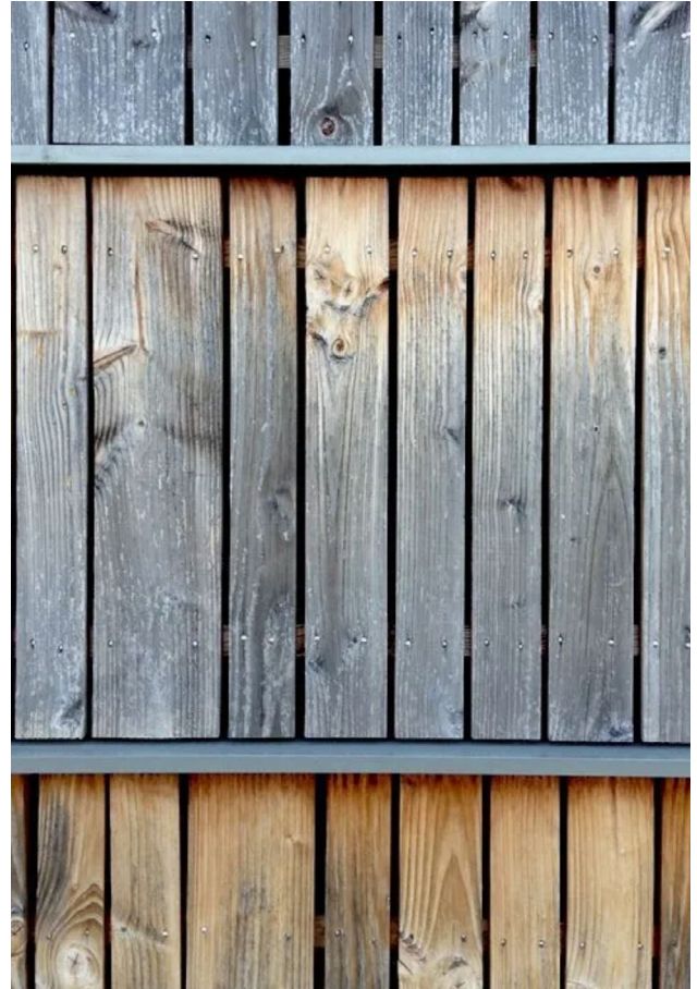
Fig. 34. (left) Wideboard vertical timber cladding of a shed in Reitdiep area, Netherlands. Photograph made by the author.
