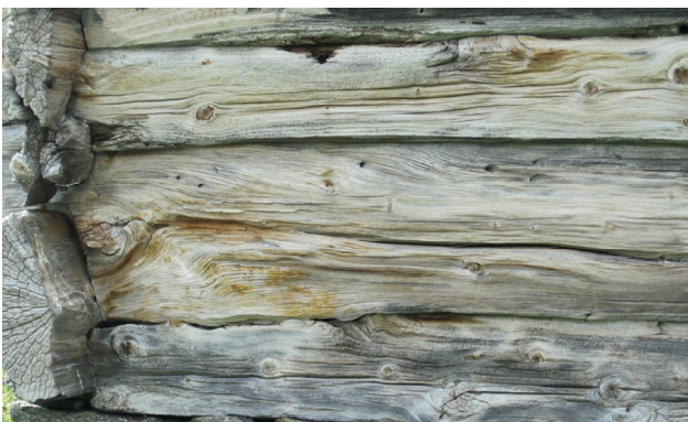
Fig. 15. (left) An old façade characterized by mechanical erosion. Vigdalen, Luster. From Weathering of unpainted wooden façades - Experience and examples (Zimmer et al., p. 23), by NIBIO/Lone Ross Gobakken, 2014.
