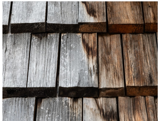
Fig. 30. (left) Horizontal cladding of overlapping boards as used in Western Norway. From Weathering of unpainted wooden façades - Experience and examples (Zimmer et al., p. 28), by Norwegian University of Science and Technology, 2014.
