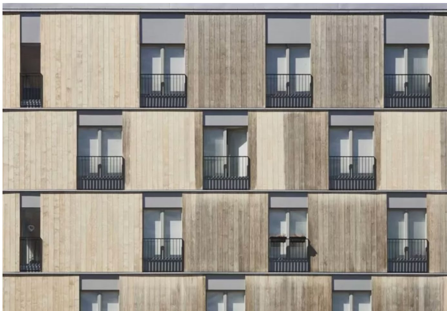
Fig. 11. Weathering of uncoated Accoya wood cladding. Wood City Block project by Anttinen Oiva Architects, Helsinki, Finland. From “Accoya”, by Accoya, n.d. ( https://www.accoya.com/accoya-weathering/ ).
