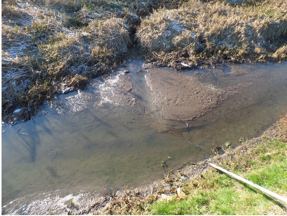
Figure 2.8: One of the boils in the west ditch (at x = 350 meter). A temperature of 9.8\text{ C}^\circ and a electrical conductivity which corresponds to 4780\text{ mg/L} has been measured here
