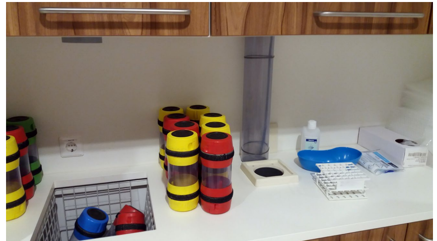
Figure 22 - Transportation pipe for sample transportation towards AKL ▲
