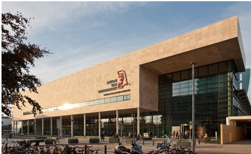
Figure 5 - Building of NKI-AVL in Amsterdam (De Ploeg, 2015) ▲
