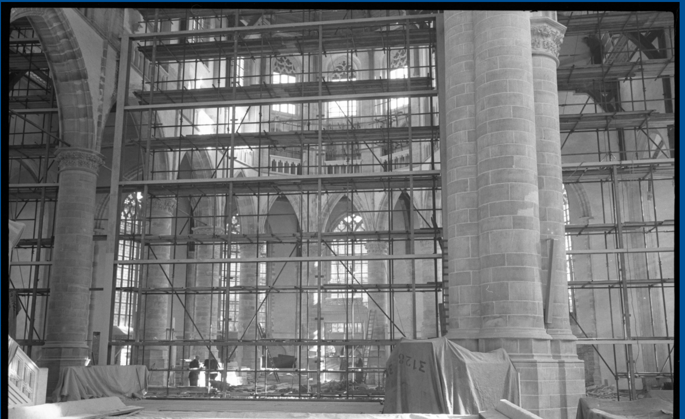
Figure 12: Restoration of the interior of the Sint Laurens church (Stadsarchief Rotterdam, 1956)
