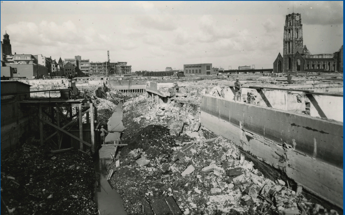
Figure 7: Overview of the Steigersgracht and surrounding area, seen from the Soetenbrug, during reconstruction work. In the background, the Delftsevaart with the building for district heating, and to the right, the damaged Sint-Laurenskerk. (Stadsarchief Rotterdam, 1941)
