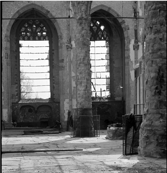
Figure 6: The interior of the heavily damaged Sint Laurenskerk shortly after the bombing on May 14, 1940. The stone pillars and some facades of the nave of the church are still standing. (Stadsarchief Rotterdam, 1940)
